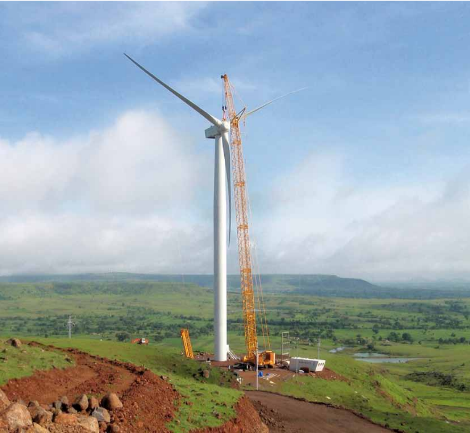
Erection of a K82 2.0 MW at Satara District, Maharashtra, India
